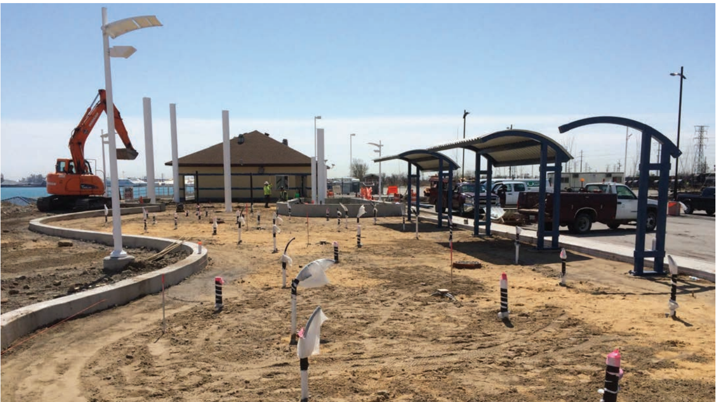
Photo 7-10. East Chicago Lakefront Park - during construction.
