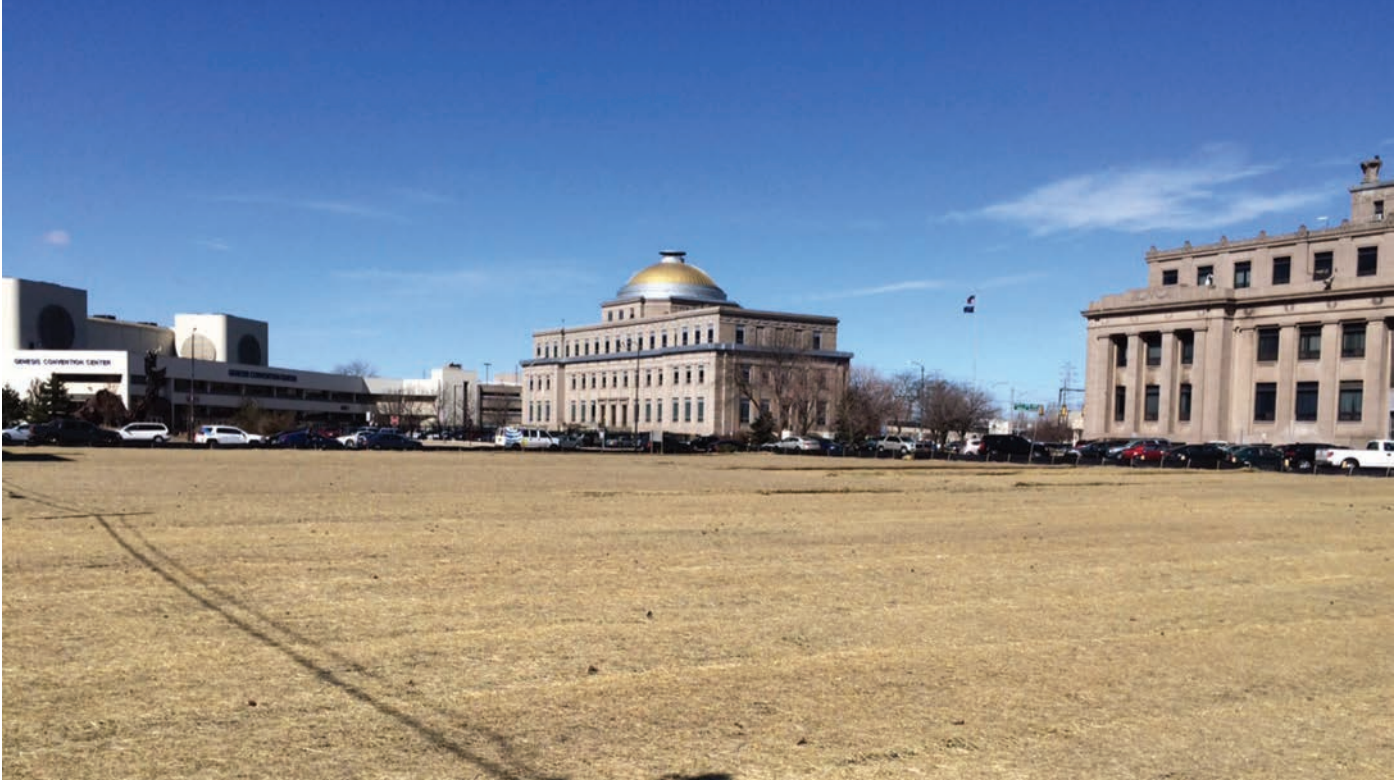
Photo 7-13. Downtown Gary Demolition Project.
