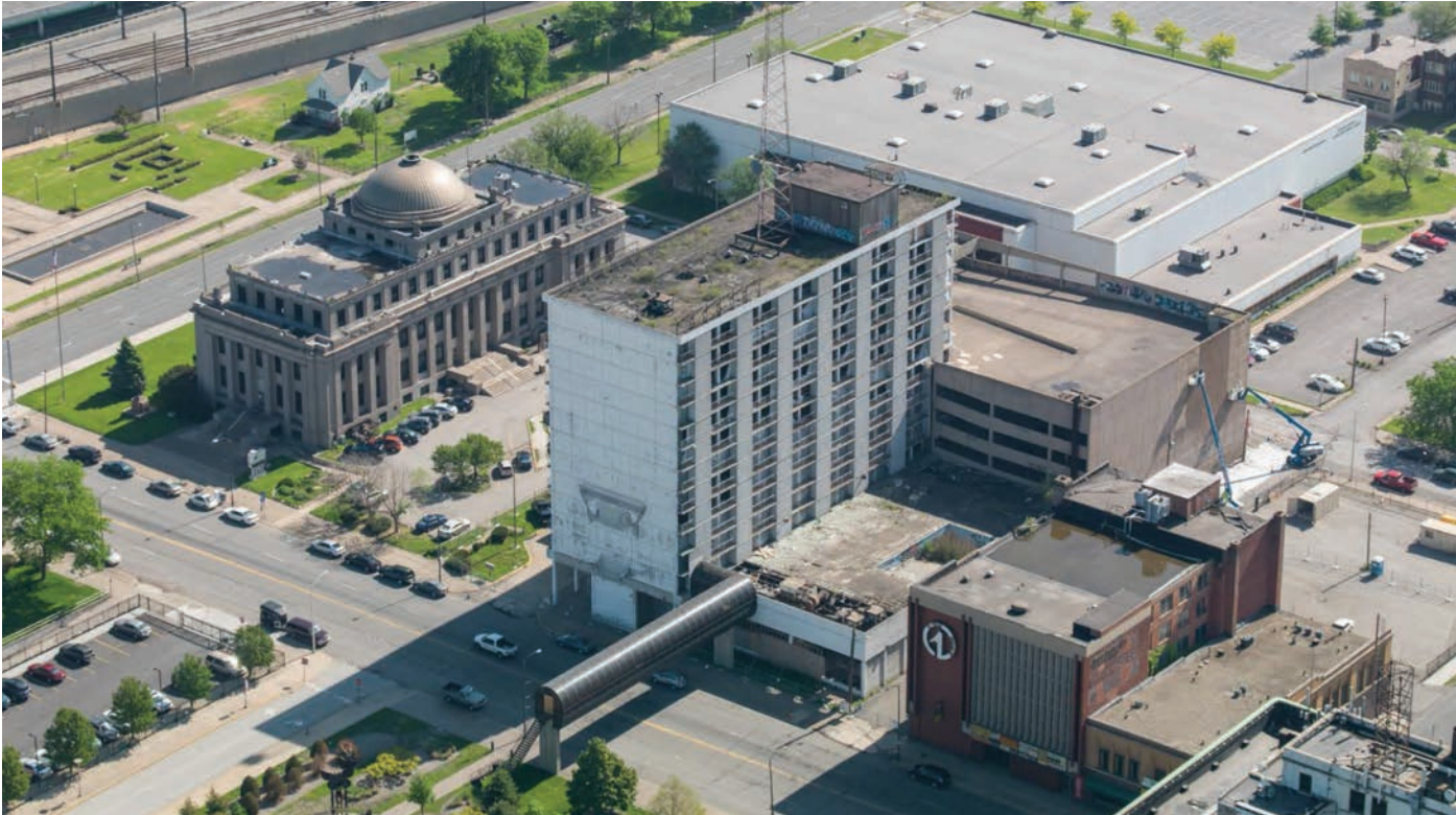
Photo 7-12. Downtown Gary Demolition Project.
