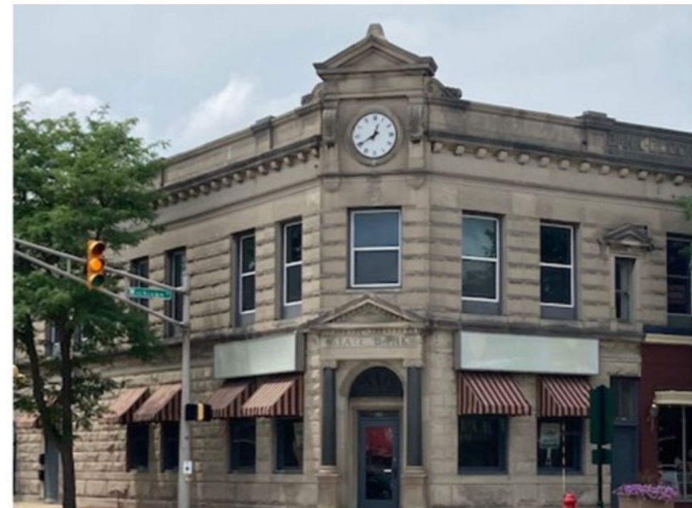
Existing Building Photo
